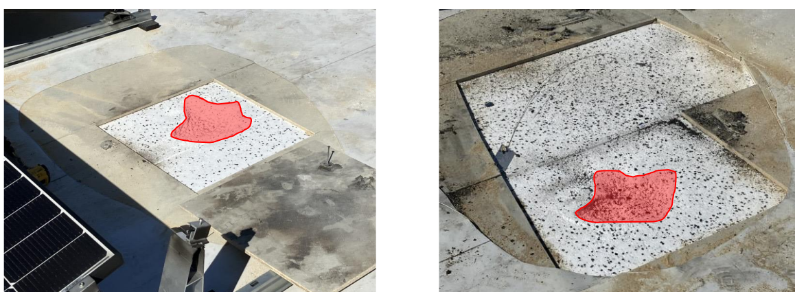
a) b) Figure 10 – Melted area of EPS under the cement-bonded particle board. a) test 5 b) test 6
