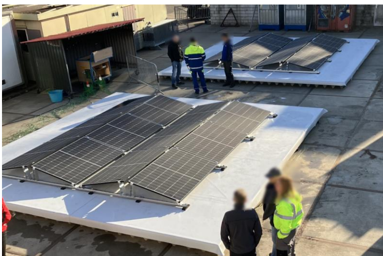
Figure 1 - Aerial view of the two roof construction build-ups used for tests 5-7.
